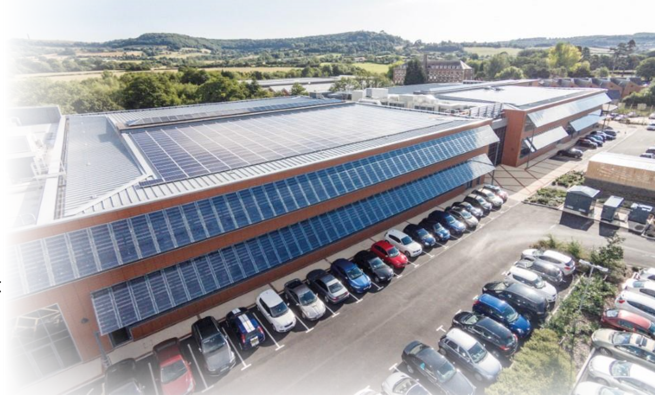
Solar panels mounted on the Renishaw Innovation Centre at our headquarters site in Gloucestershire, UK
