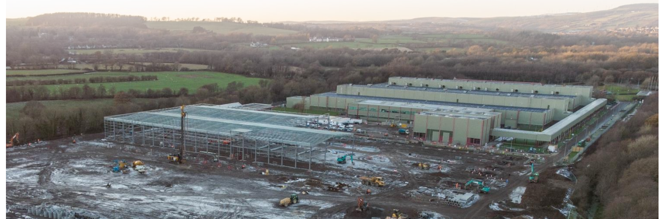
Progress on Miskin manufacturing expansion (December 2022)
