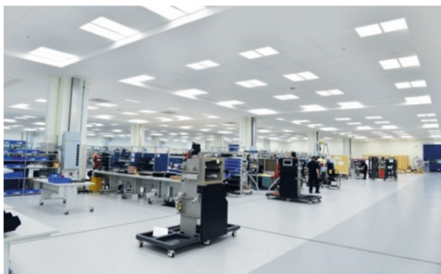
LED lighting has reduced energy demand for lighting in the UK by around 80% (image of assembly area at Miskin).
