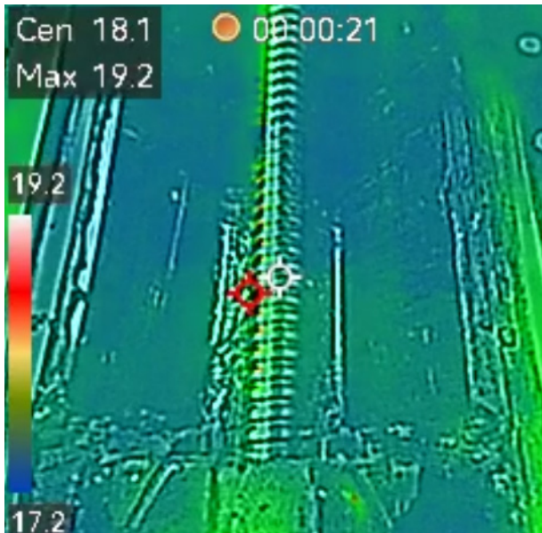
Figure 3: This thermal image (thermogram) shows the machine at room temperature. It is apparent that the ballscrew is about the same temperature as the background reading for the machine.
