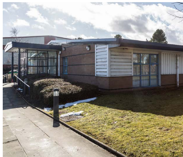
Apex's facility in Loanhead
